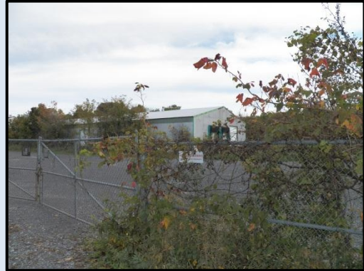
Existing warehouse at the former W.R. Grace Company Site on Dunn Rd in Brutus
