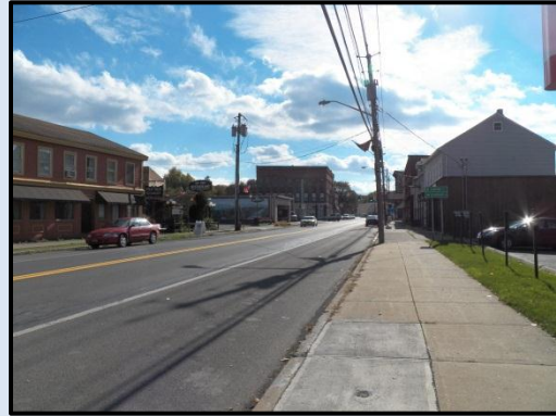
Existing pedestrian realm along State Route 34 in the Village of Weedsport. There is no buffer between the pedestrian on the sidewalk and the truck traffic on the street. A more inviting streetscape should be developed.
