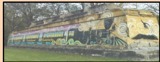
Mural on the side of the former railroad abutment on State Route 31 east of Aqueduct Park
