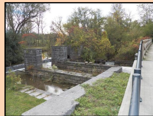
Remnants of the old aqueduct, Cold Springs Brook flowing through it, and the pedestrian bridge/bike path which goes over the creek out to Port Byron
