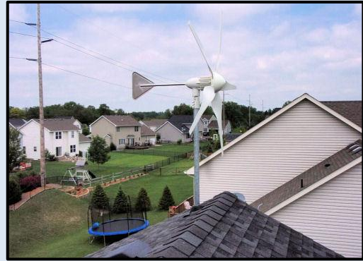
Example of a small scale residential wind energy generation system.
