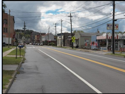
Existing commercial core of the community along State Routes 34 & 31
