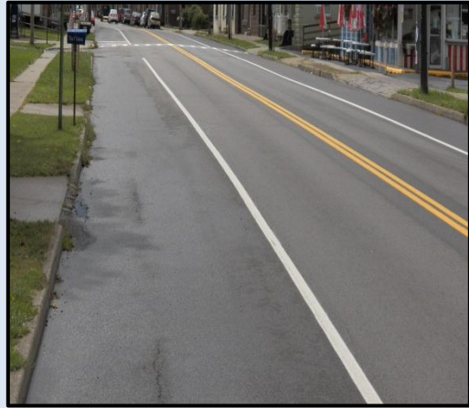
Existing on-street parking along State Route 34- no striped spaces
