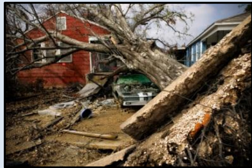
Property damage from a natural disaster
