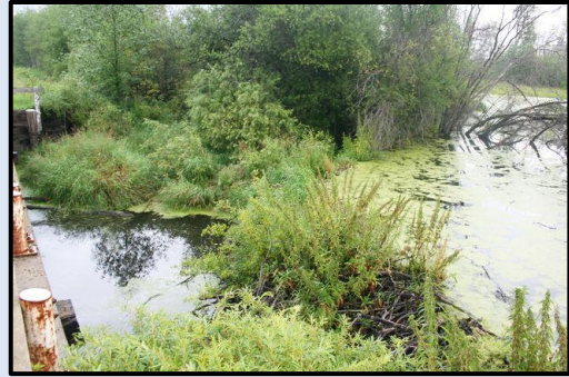
Flooding caused by a beaver dam
